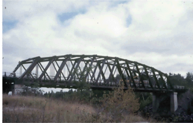
Fig. 6.1 The Sioux Narrows bridge in Ontario, Canada which was believed to be the longest-span timber bridge in the world
